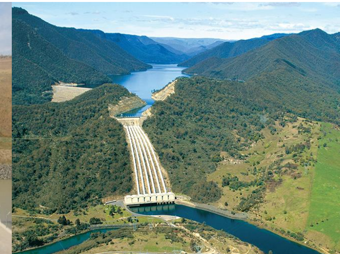
Credit – Hydroreview 2,200 MW Snowy 2 Open Loop PSH Under construction (2029), Australia
